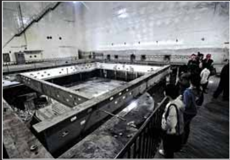
The nuclear reactor hall, as large as a soccer field, forms the core of the underground plant.
